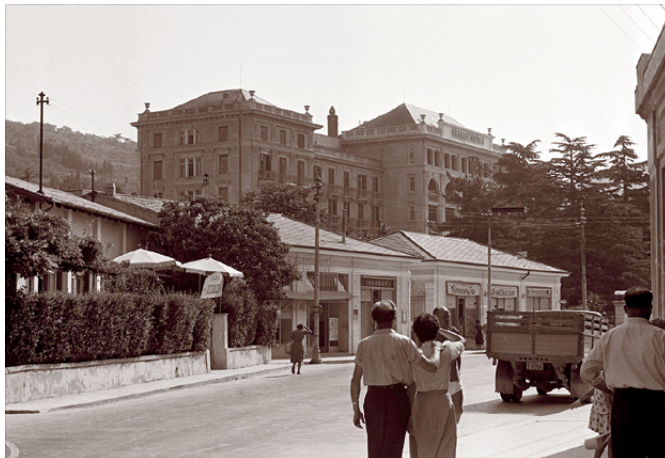
Figure 6: Palace Hotel in 1957. (Source: Večer).
